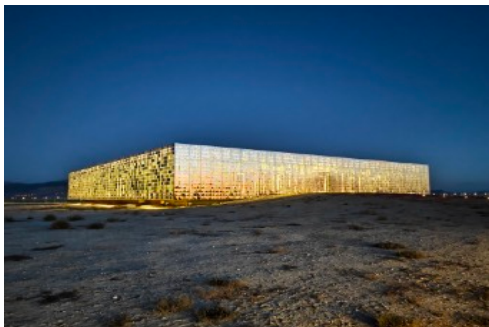
Karapınar Scada Building - Konya TR
